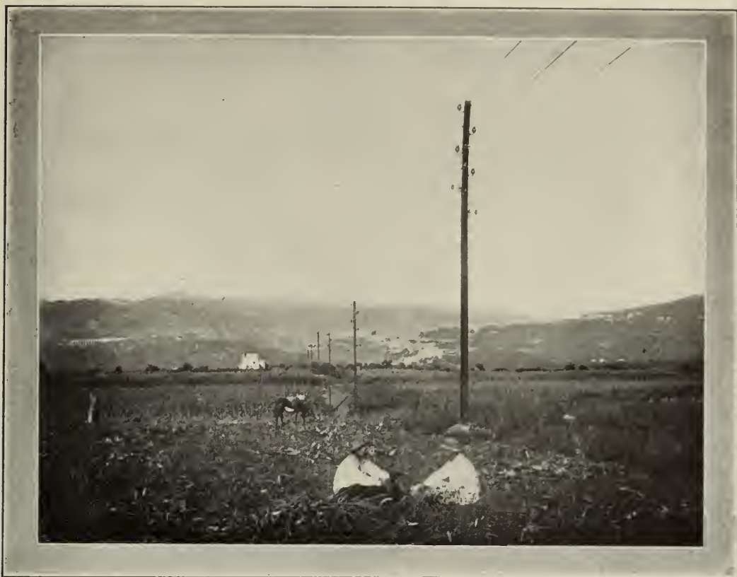
FIG. 10. THE TRANSMISSION LINE ON THE CAMPAGNA ROMANA.
